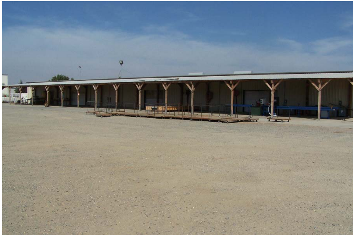
View from rear of building
